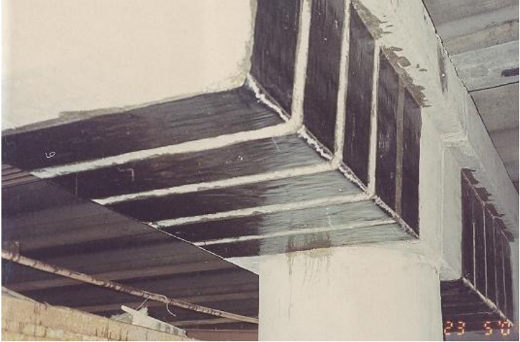
Shear strengthening
