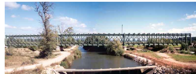
Bridge over the Soure river
