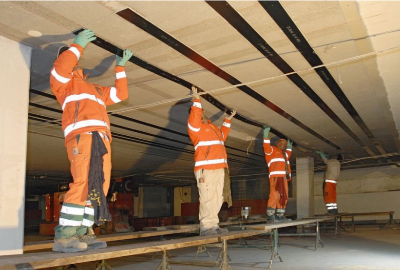
Flexural strengthening
